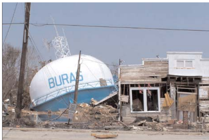
Water Tower in Buras, LA Photo: Louisiana Department of Environmental Quality
