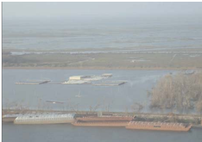
Mississippi River Levee in Front of Plaquemines Parish Prison Photo: Louisiana Department of Environmental Quality
